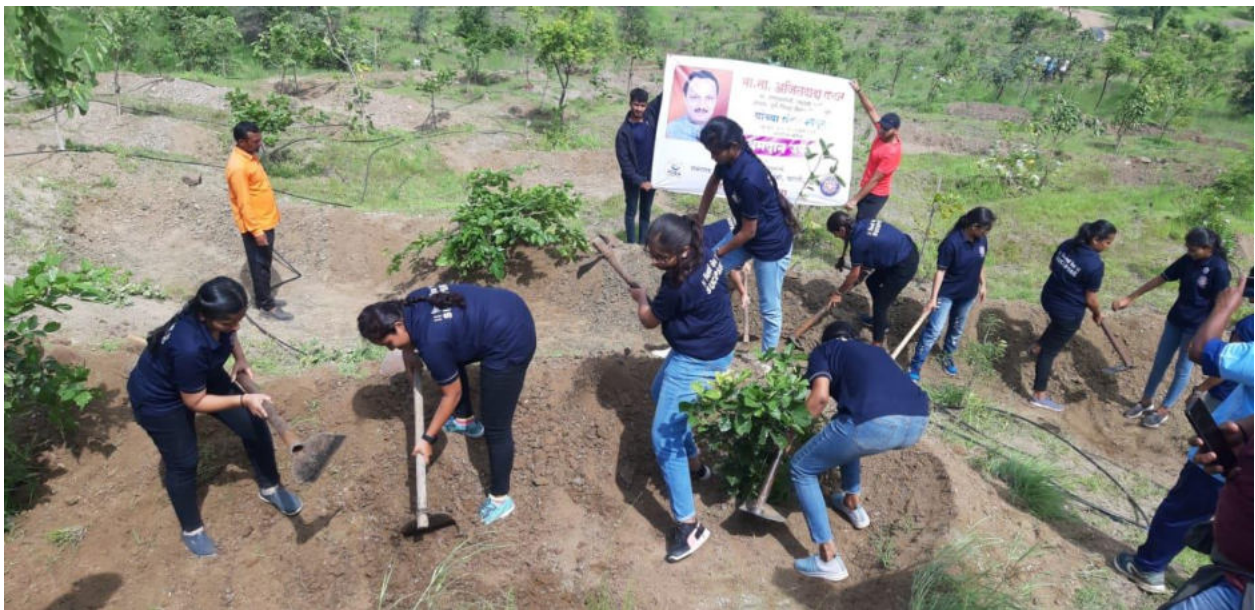
Work for the purpose of water conservation and water horizontally by digging continuous counter trenches(CCT) on the Bakori hills.
