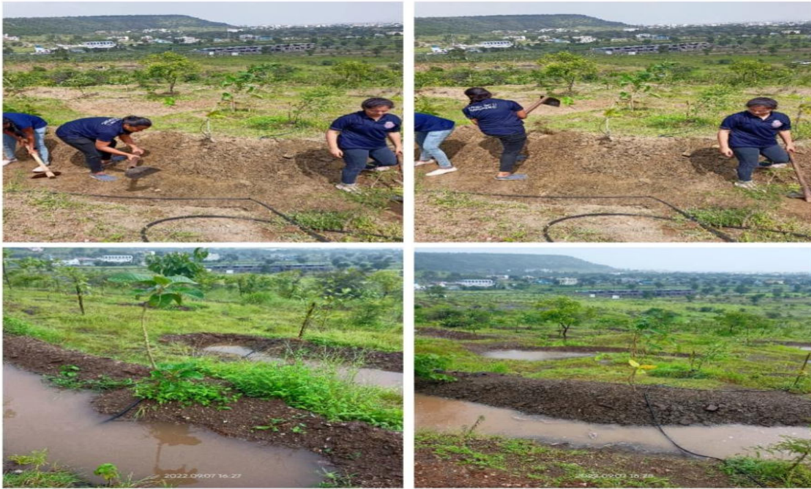
Impact of work done for the purpose of water conservation by digging continuous counter trenches(CCT) on the Bakori hills.
