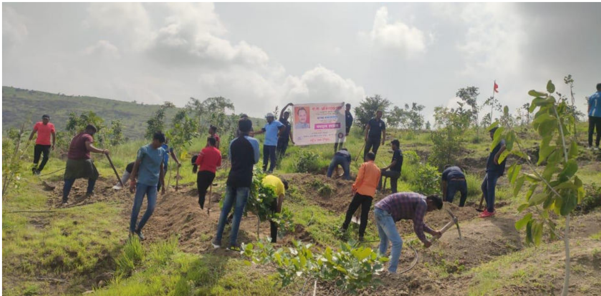
Work for the purpose of water conservation and water horizontally by digging continuous counter trenches(CCT) on the Bakori hills.
